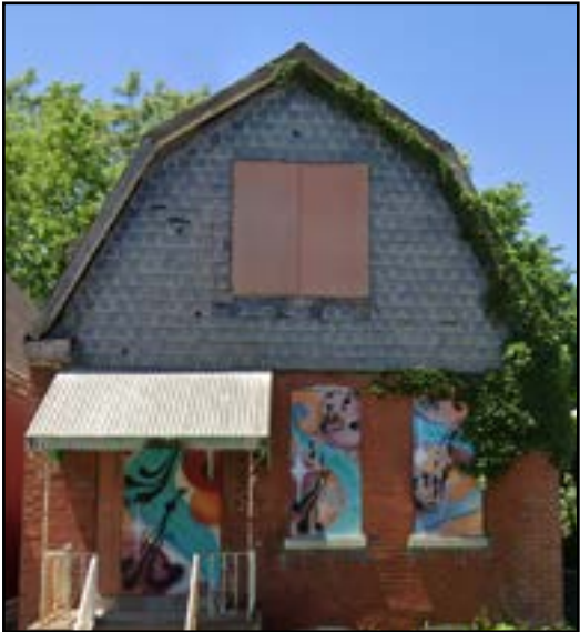
GAMBREL ROOF W/ ORIGINAL SLATE
